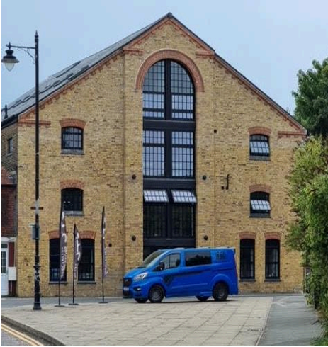
48 Ferry Road following Conversion of Night Club
